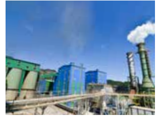
Bolu, Göynük Thermal Power Plant
