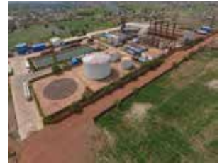
Madagascar Heavy Fuel Oil Power Plant
