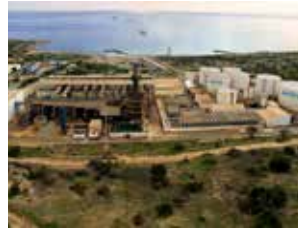
TRNC Heavy Fuel Oil Power Plant
