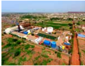
Republic of Congo Natural Gas Power Plant
