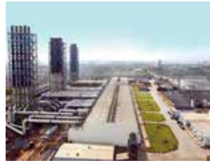
Ghana Heavy Fuel Oil Power Plant
